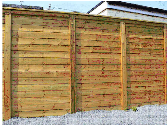
Image of proposed 2m high acoustic fence
